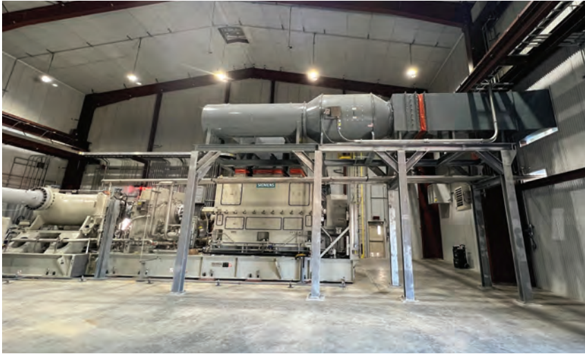
Bi-Con constructed the two-unit electrical driven compressor for the natural gas compressor station project. The unit was built and manufactured offsite, and Bi-Con installed it, connected all the piping and electrical to make it operational. Location is confidential.
