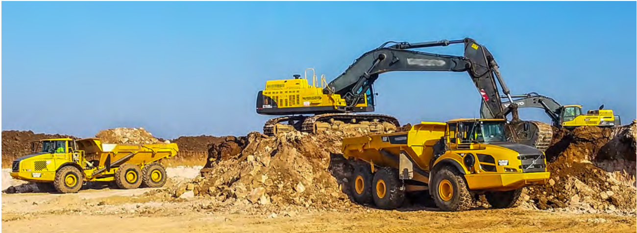
Wondra Construction, a heavy civil contractor involved in wetland restoration, large manufacturing projects and road construction, performs mass grading on a jobsite.
