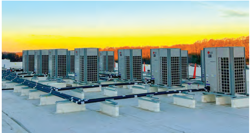
D.J. Wagner Heating & Air Conditioning Inc. was hired as the mechanical contractor on the Northeast Regional Center project in Newtown Square, Pennsylvania, to provide and install an energy recovery unit, two rooftop units, 14 variable refrigerant flow systems with 80 indoor air handlers, and all associated refrigerant piping, condensate piping, ductwork, insulation and controls. This project is anticipated to be completed in the winter of 2026.
